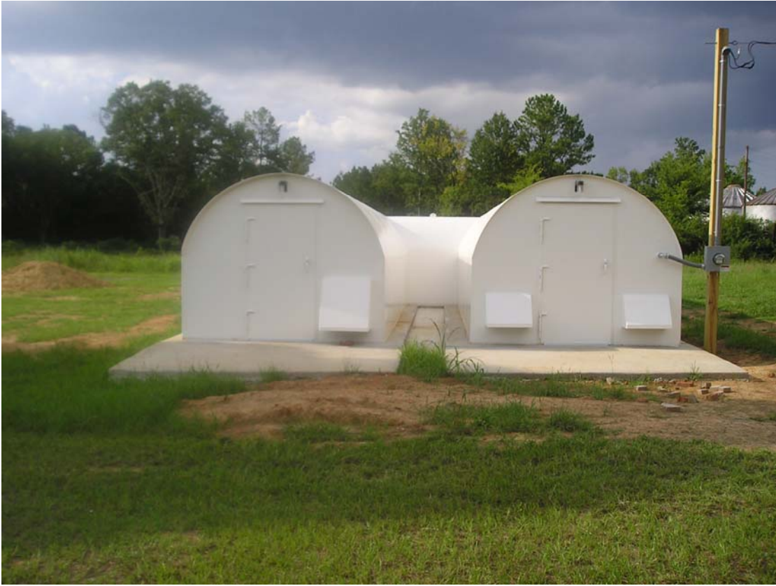
Vincent Community and Civic Center Community Storm Shelter 5384 Highway 62, Vincent. The shelter is located east of Vincent at the intersection County Road 62 and Gorman Park Road.
